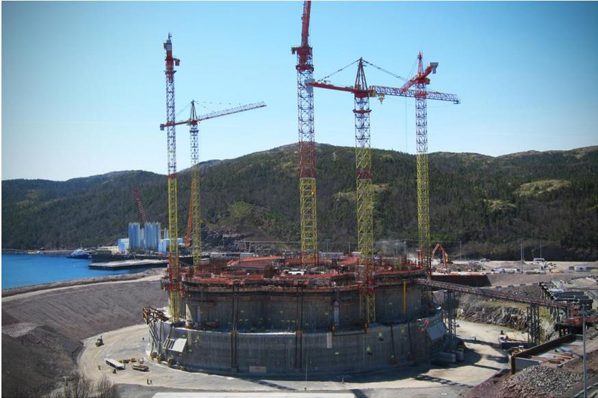
**Figure 6: Construction of the Hebron concrete GBS at the Bull Arm site, Newfoundland (Photo: ExxonMobil Canada)**
