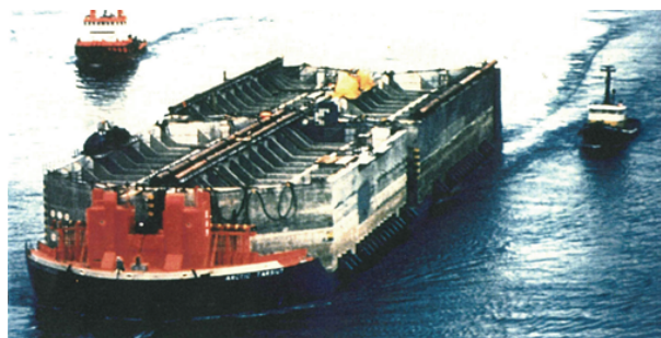
Figure 18b: Tarsiut Caissons deploying from Vancouver to Beaufort Sea (Photo: B. Maddock)
