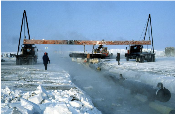
Figure 15a: Laying pipe through ice trench (Photo: D. Masterson)
