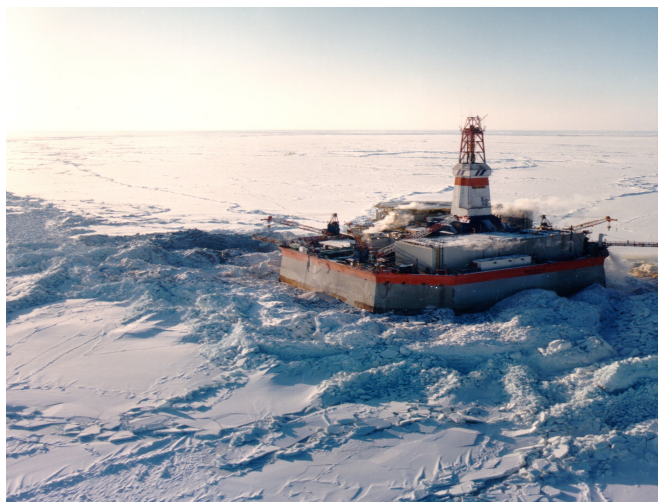
Figure 1-21. The Molikpaq Caisson 70
