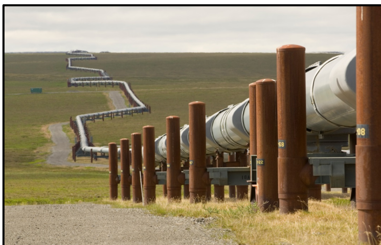
Figure 1-26. Trans-Alaska Pipeline Zigzag Design 78
