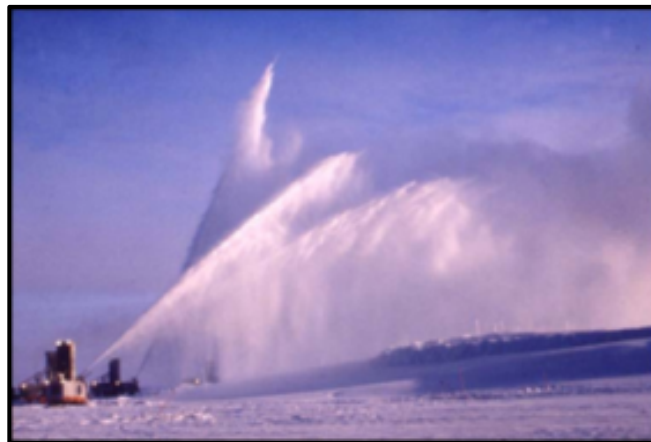
Figure 1-30. Spray Ice Island Construction
