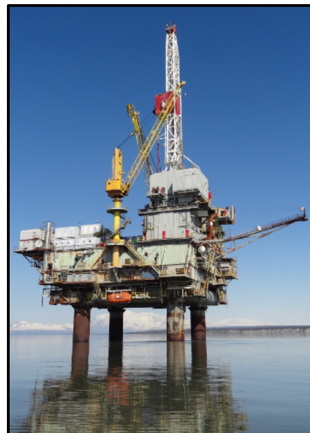
Figure 1-28. Cook Inlet Platform with Tower Type Jackets
